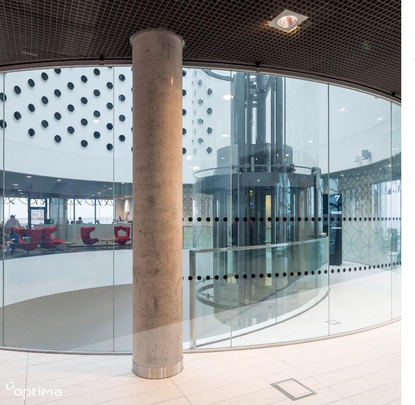
The unique design of the building's interior required Optima to engineer and install a number of bespoke solutions. This included the curved fire screens, all of which were different with specific design requirements.
